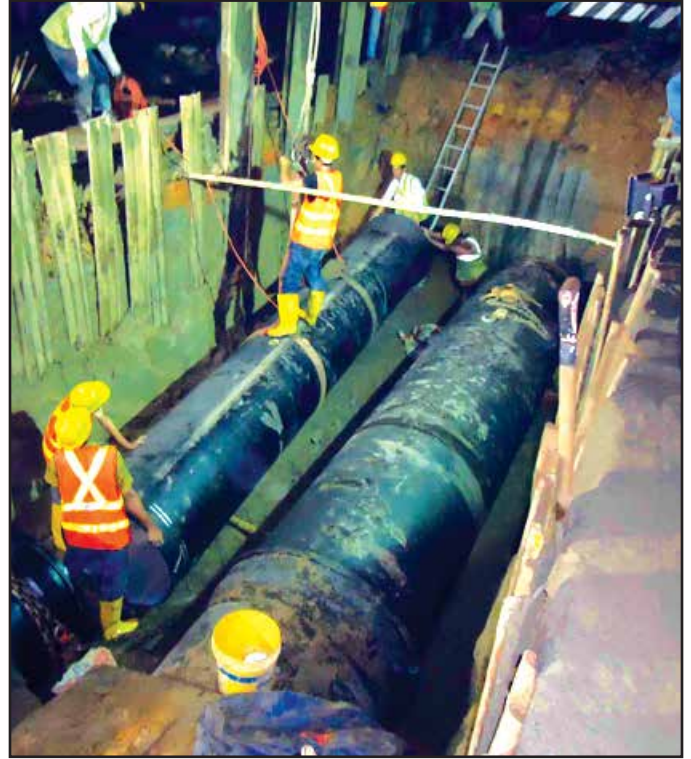
Dual Pipe Laying
