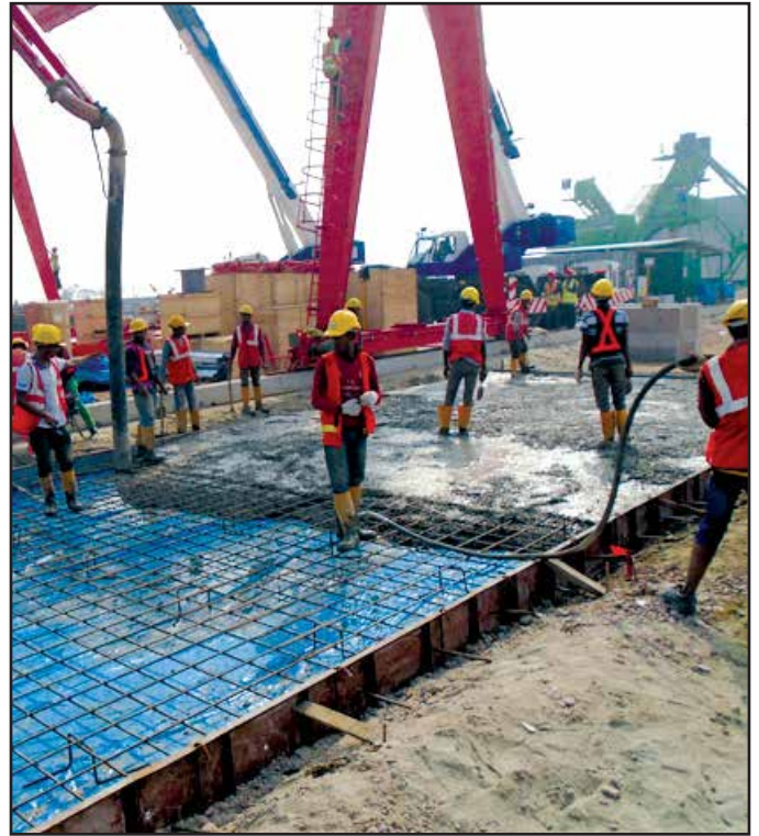
Construction of 6m Wide RCC Road at Casting Yard CP-03-04
