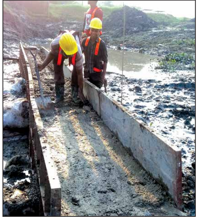
Concreting Work for Mushurikhola Canal Crossing
