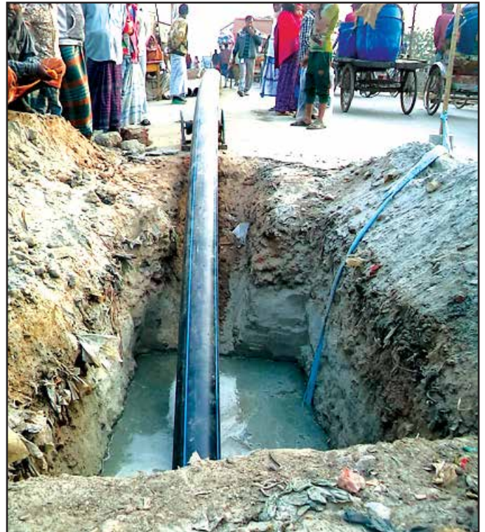
Pulling HDPE Pipe by HDD Machine
