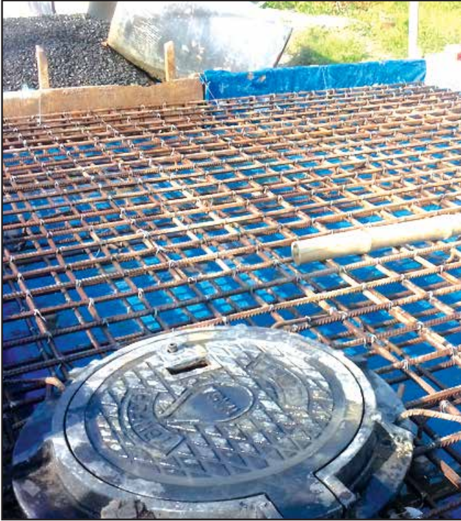
Bulk Water Meter Chamber Roof Slab
