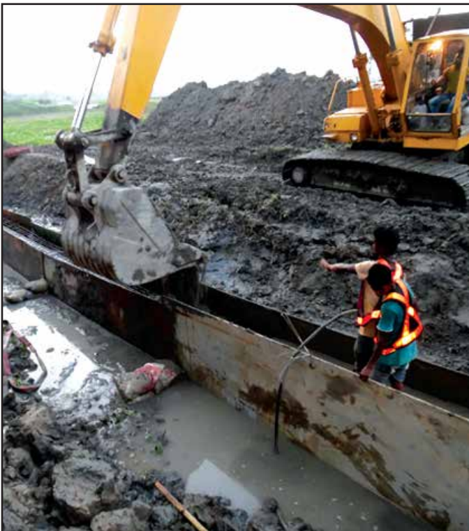
Excavator at Work for Mushurikhola Canal Crossing
