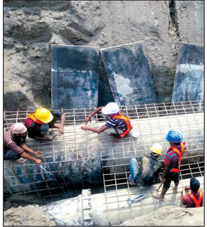
Rebar Work for Surrounding Concrete
