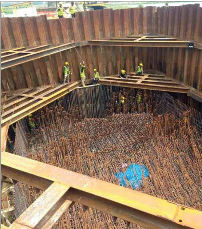
Shear Link and Rebar Work for Balance Cantilever Pile Cap
