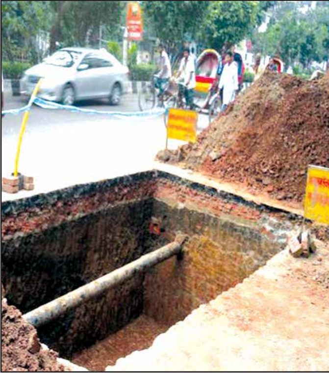
Earth Excavation for BWM Chamber Work
