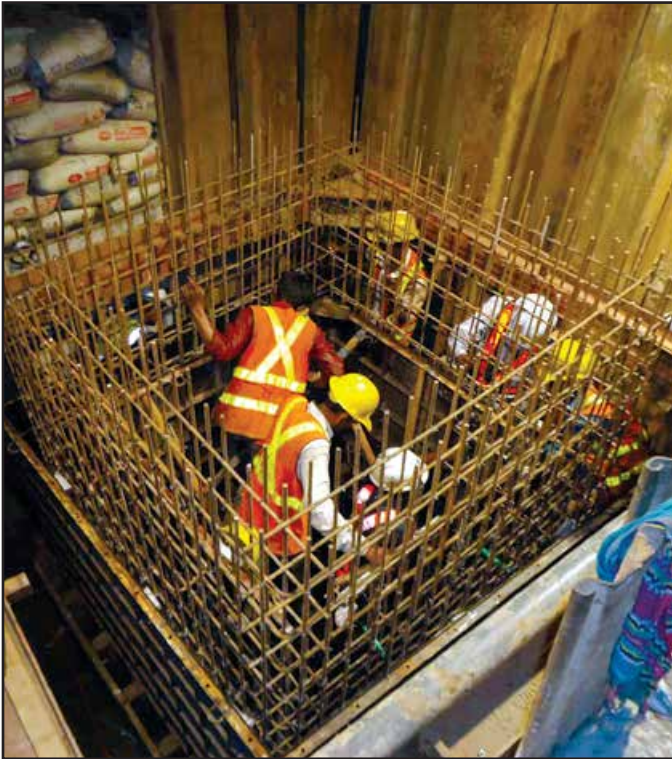
Shuttering of Butterfly Valve Chamber
