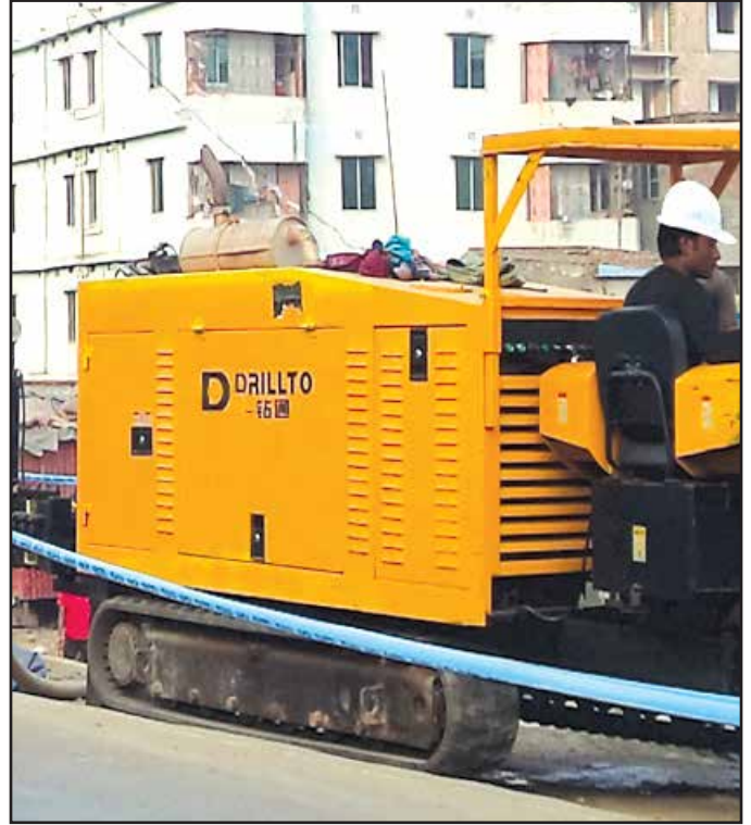
During HDD Work at Beribaad Road
