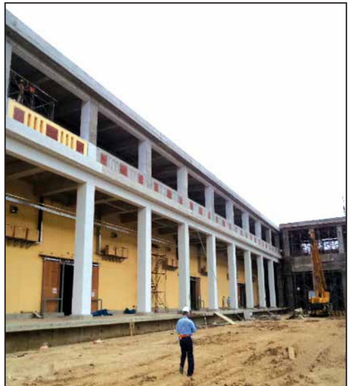
Construction of Truck Yard in Progress
