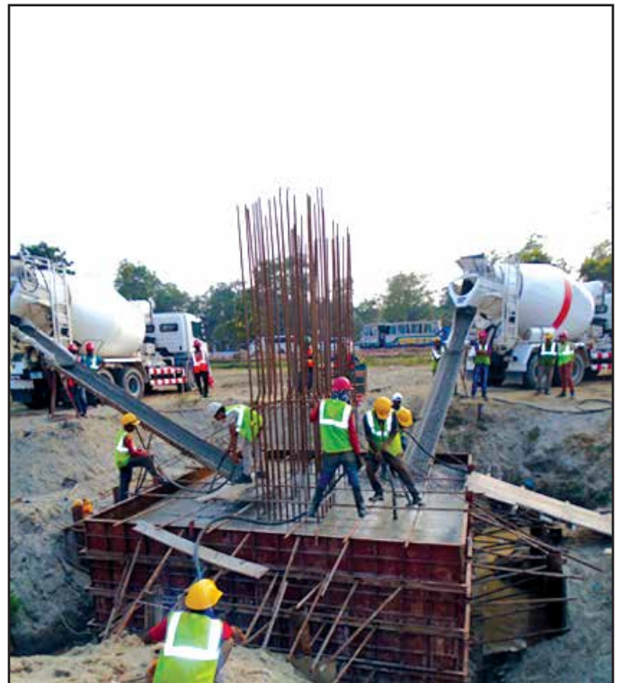
Concreting of Pilecap
