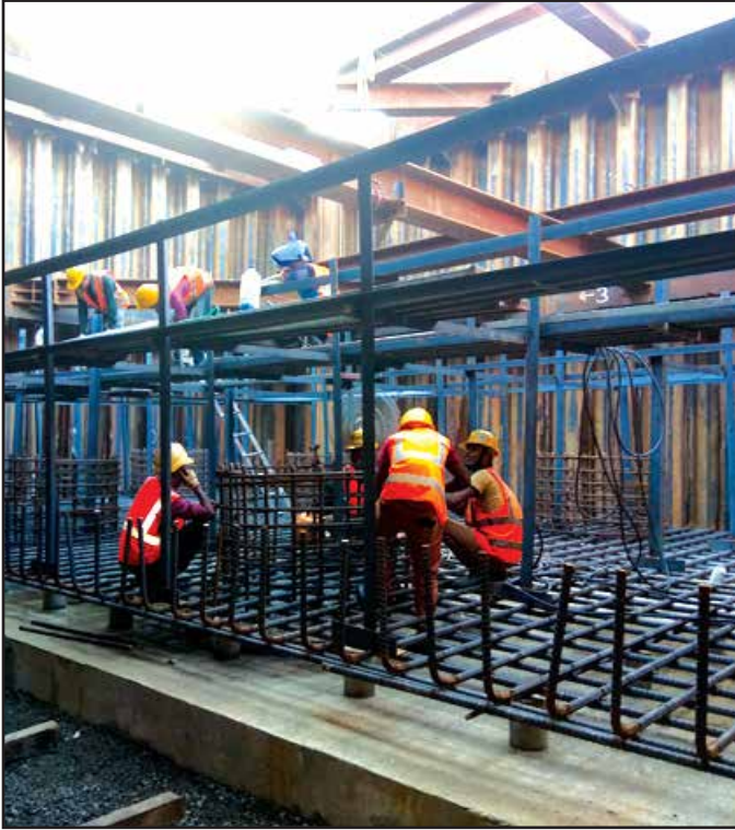
Pier- 11 Base Rebar Fixing & Angle Frame Installation for Final Layer
