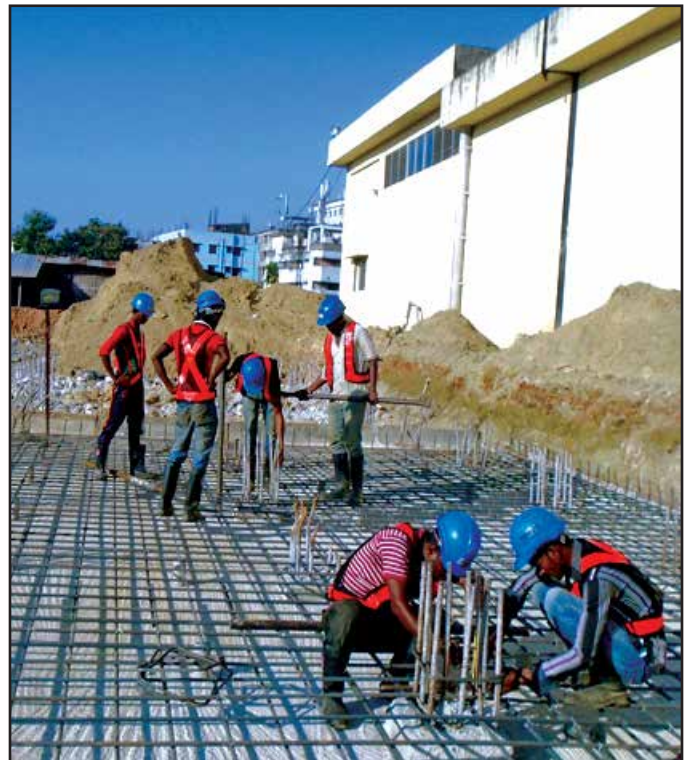
Rebar Work for Base Slab of Reservoir
