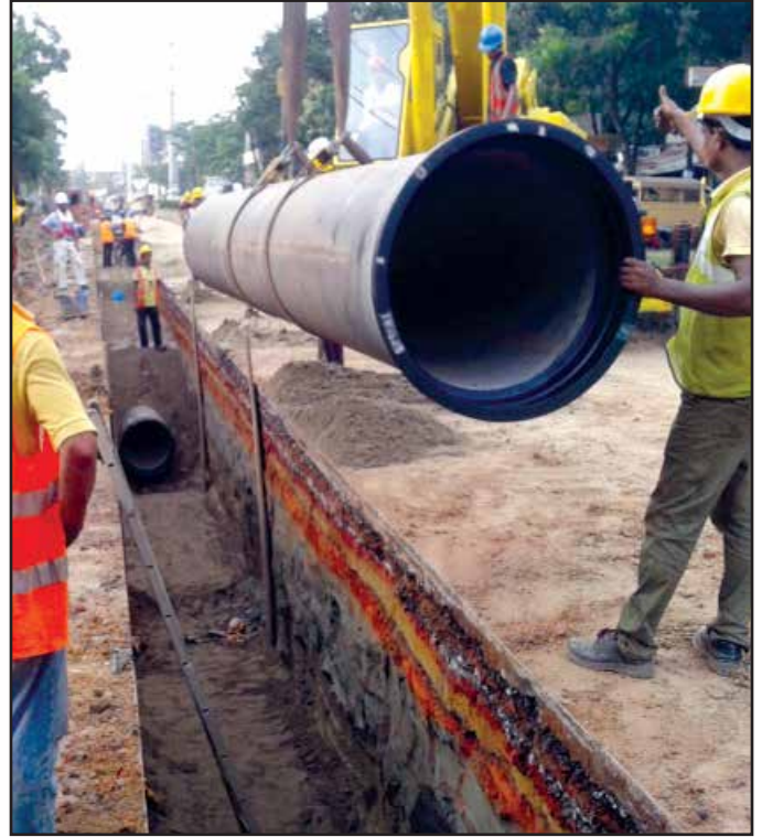
Pipe Laying in Progress
