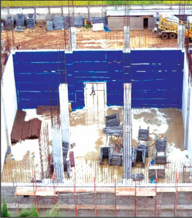
Construction of Ground Floor Wall & Column Completed
