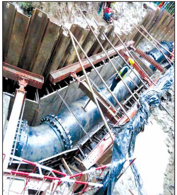
Pipe Laying with Restrained Joint at Divert Crossing
