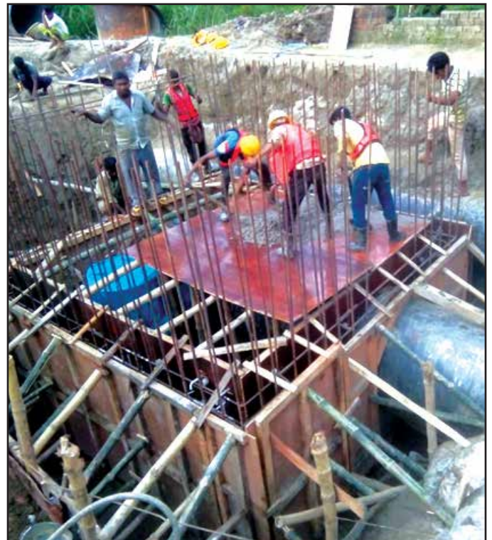
Bulk Water Meter Chamber Wall Concreting
