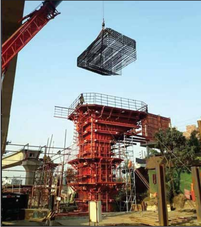
Asymmetric Pier Head Rebar Case Installation Work
