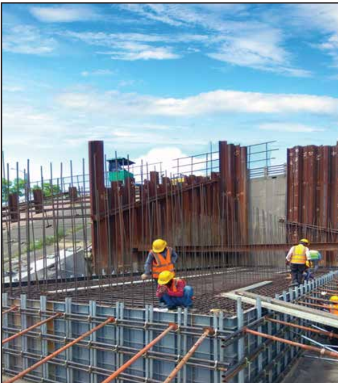
Rebar & Formwork for Abutment-2 at Meghna Site
