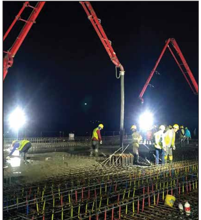
Deck Slab Concrete Work at CP-03 (P16 to P22)
