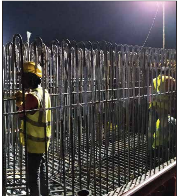
Portal Pier (Cross Beam) Rebar Work
