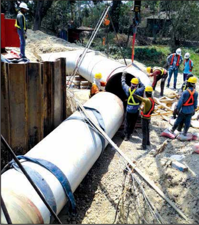
Pipe Joining at Overpass Section
