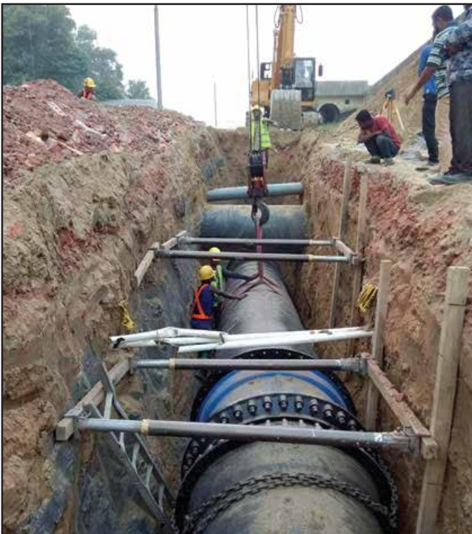
DI Pipe Laying Work (During Installation)
