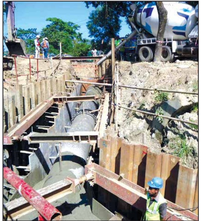
Protection Concreting at Divert Crossing
