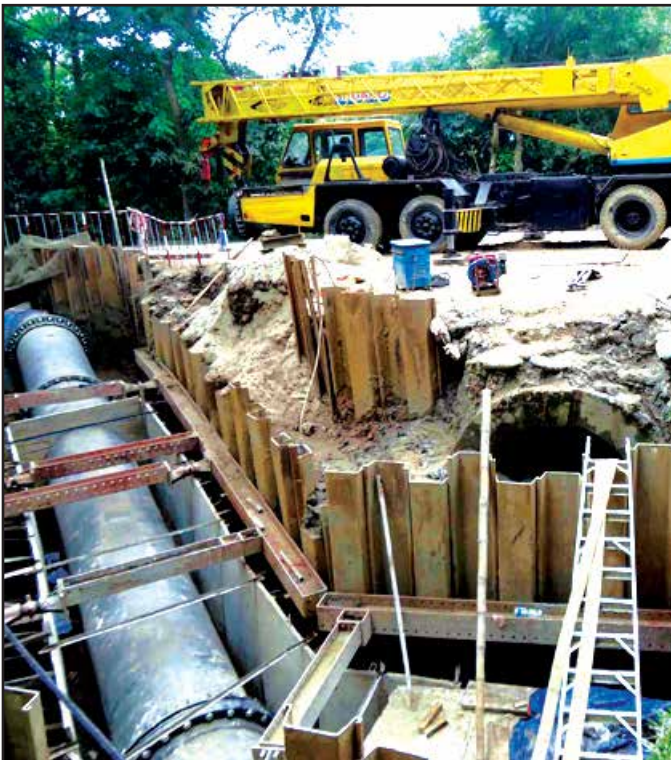
Divert Crossing with Restrained Joint
