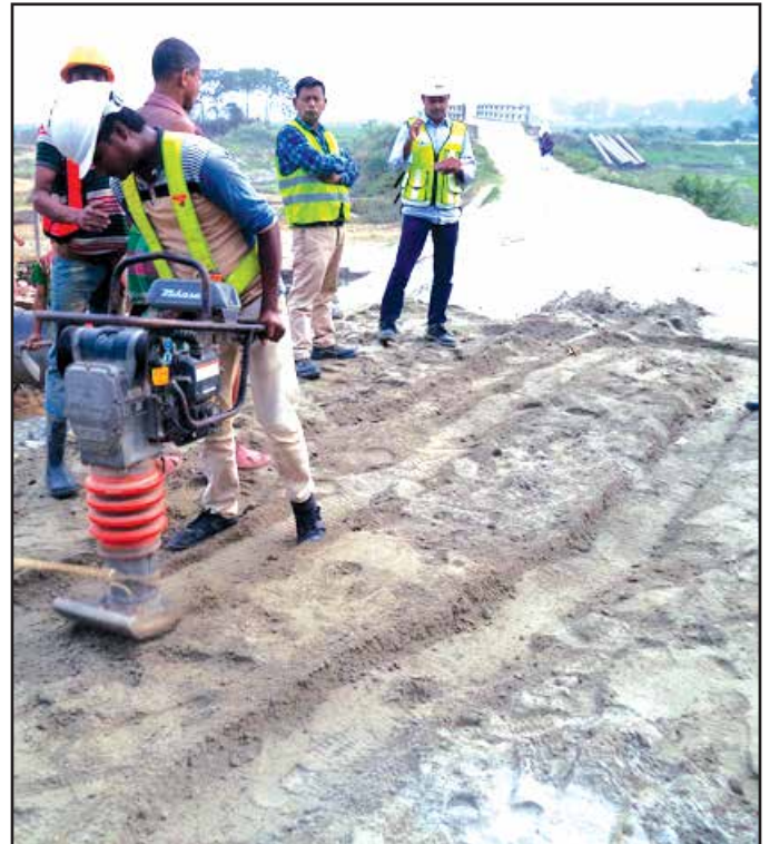
Sand Compaction Work with Tamping Rammer after Pipe Laying
