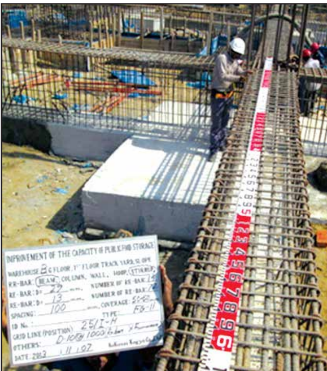
Construction of Ground Beams
