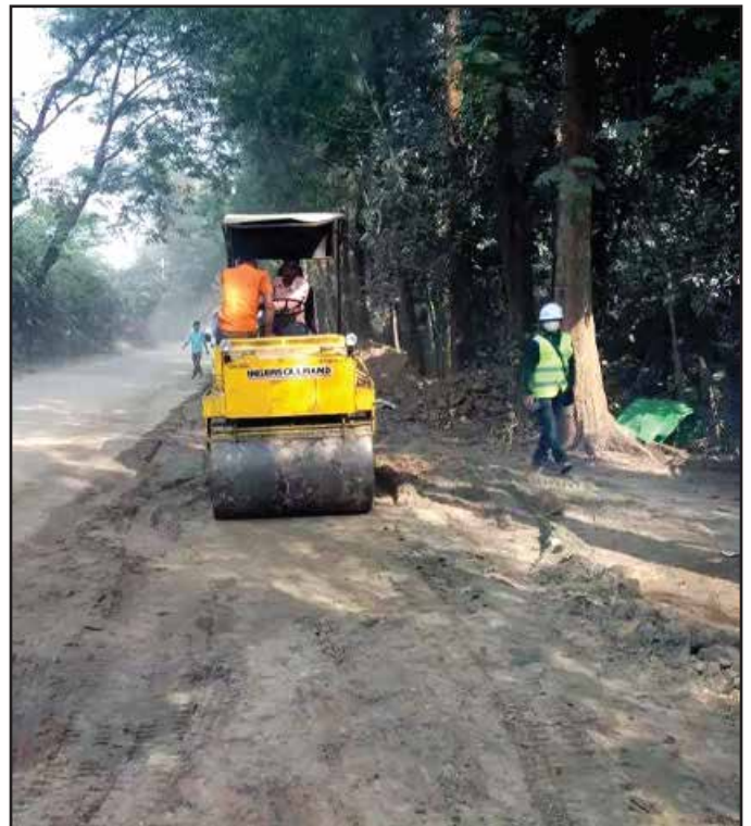
Road Leveling Work Using Road Roller
