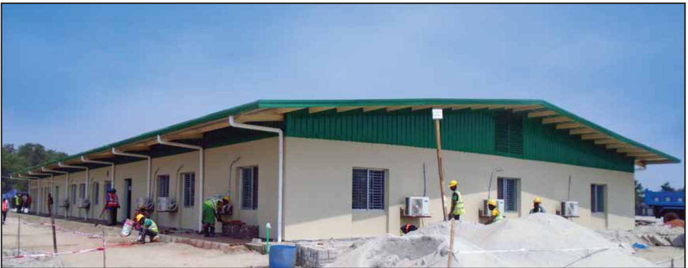
Completed Site Office of OSJI JV
