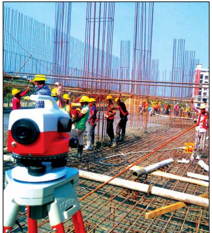
Level Checking during Reservoir Base Concreting
