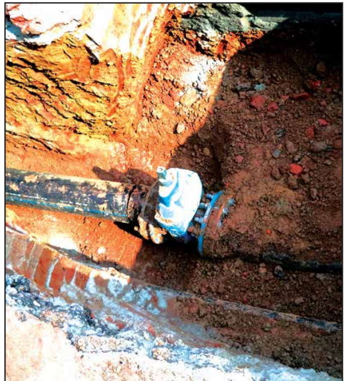
Gate Valve Setting at Junction Point
