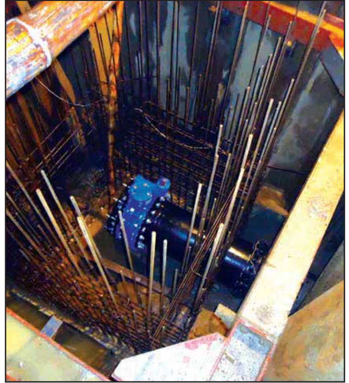
Installation of Butterfly Valve
