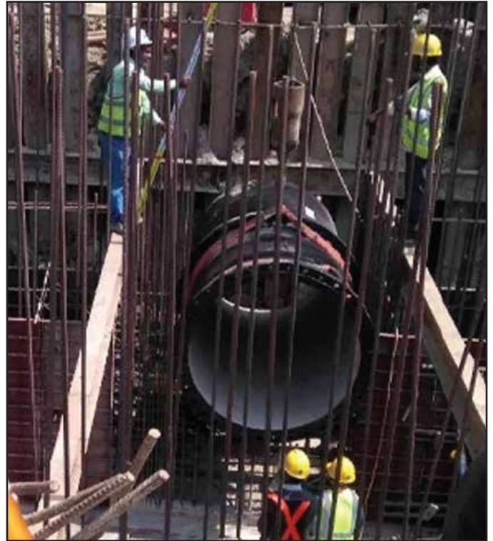
Installing Outlet Pipe at Outlet Pit
