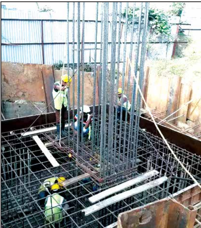
Rebar & Formwork for Pilecap
