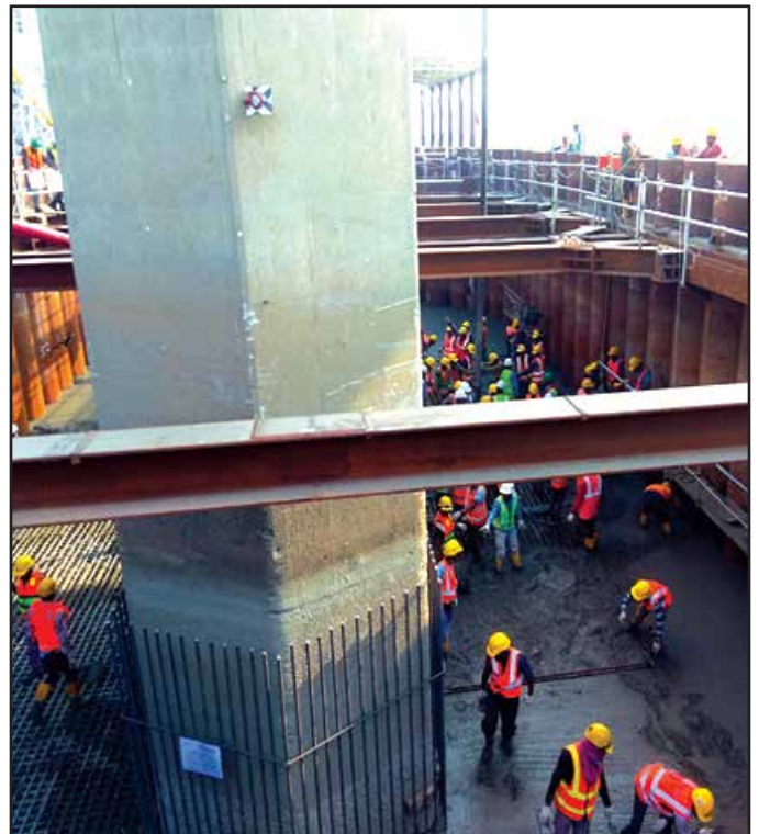
Pier-10 Final Base Layer Concreting
