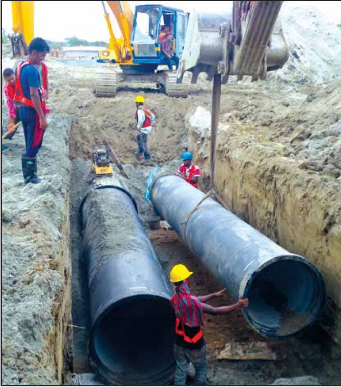
Dual Pipe Laying Work
