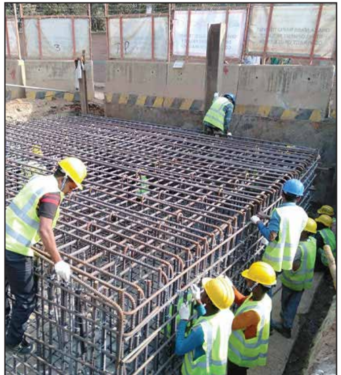
Pile Cap Rebar Binding Work
