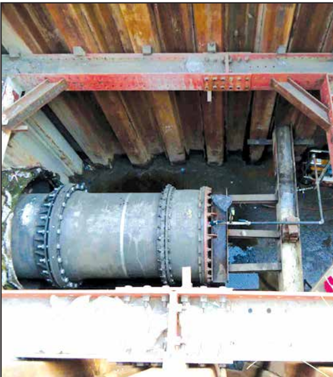
Pressure Test at Railway Undercrossing
