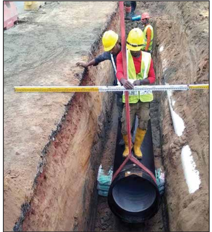
DI Pipe Laying and Leveling Work (During Installation)
