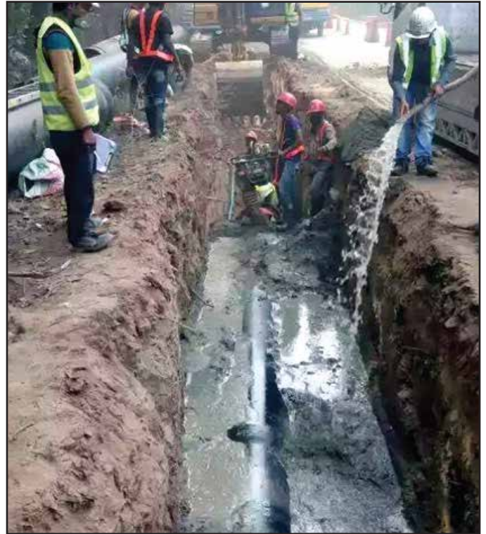
Spraying Water During Backfilling
