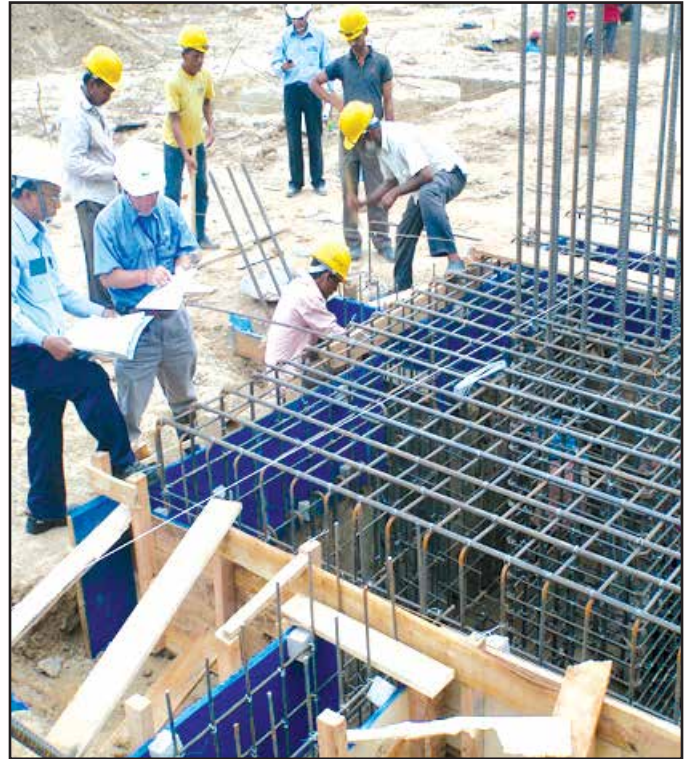
Installation of Rebar & Formwork for Pilecap & Column
