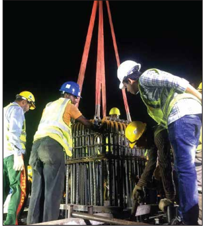
Construction of Seismic Buffer
