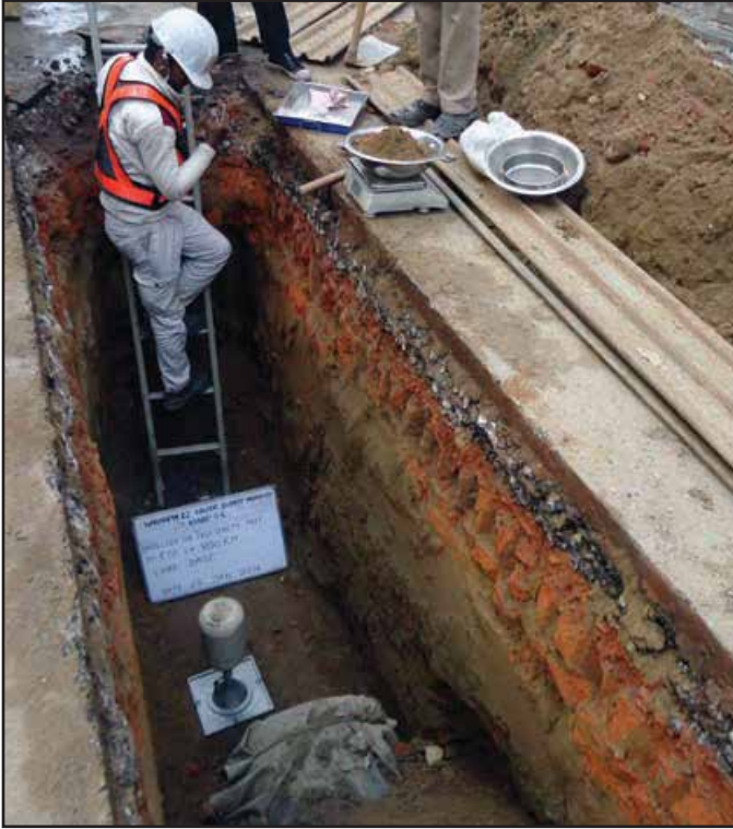
FDD Test-Step-2 of Prepared Bed
