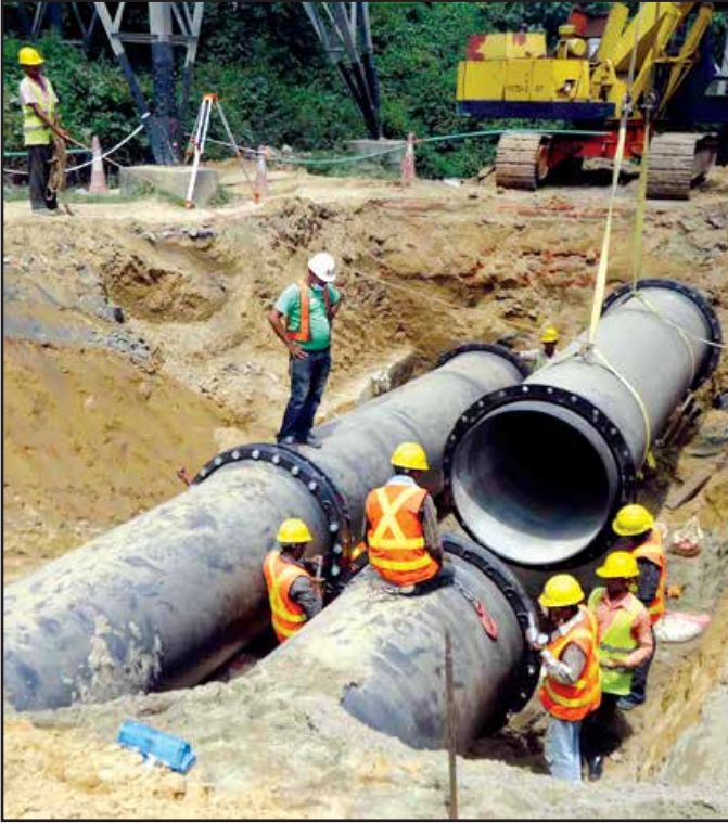
Double Line Pipe Laying Work
