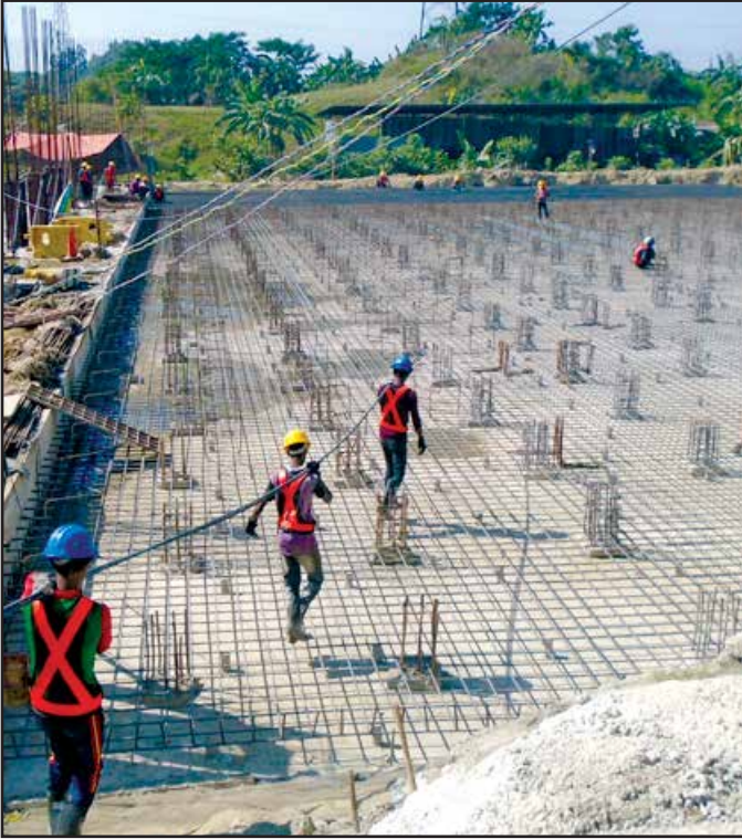
Base Slab Rebar Work in Progress
