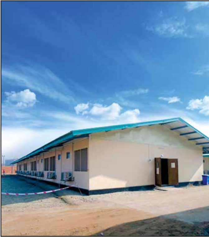
Construction of Thai Camp at Casting Yard CP-03-04
