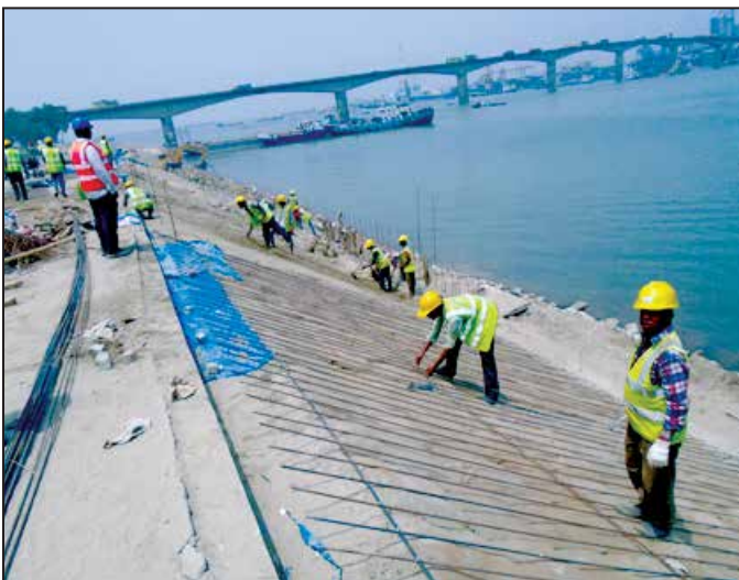
Slope Protection Work at Jetty Area
