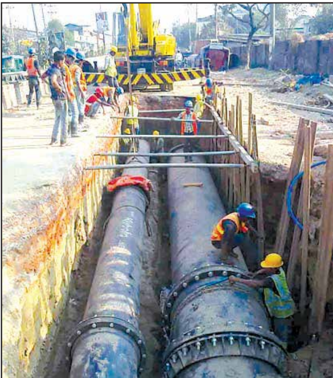
Installation of Double Line Transmission & Distribution Pipes
