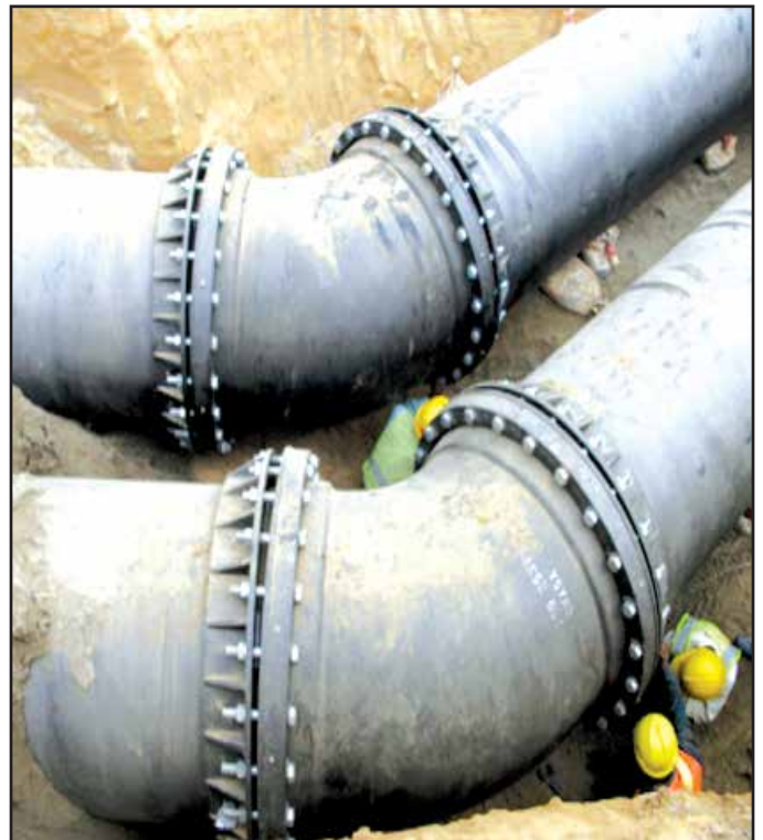
Setting of THL Joint with Bend
