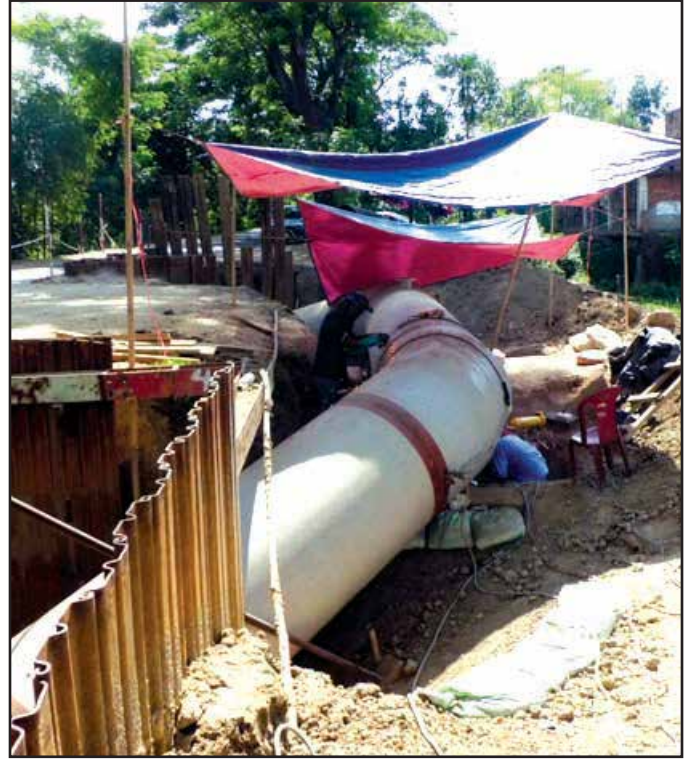
Pipe Laying Work on a Culvert
