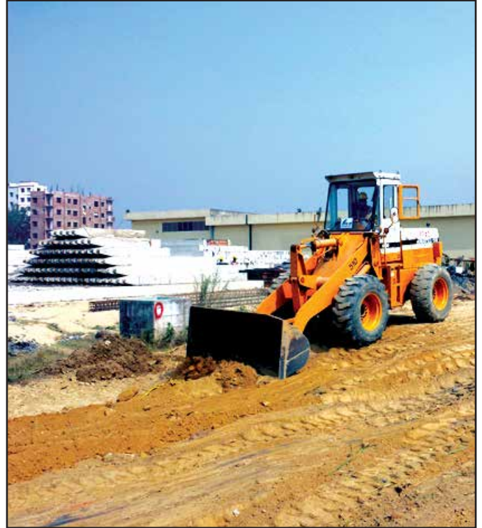
Removing Debris using Payloader
