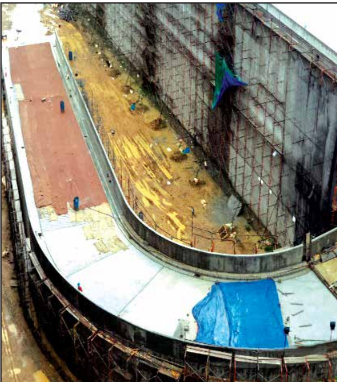
Construction of Access Ramp to Level- 2
