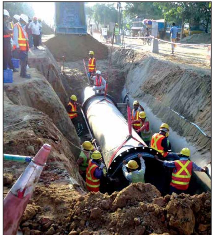
Pipe Laying Work
