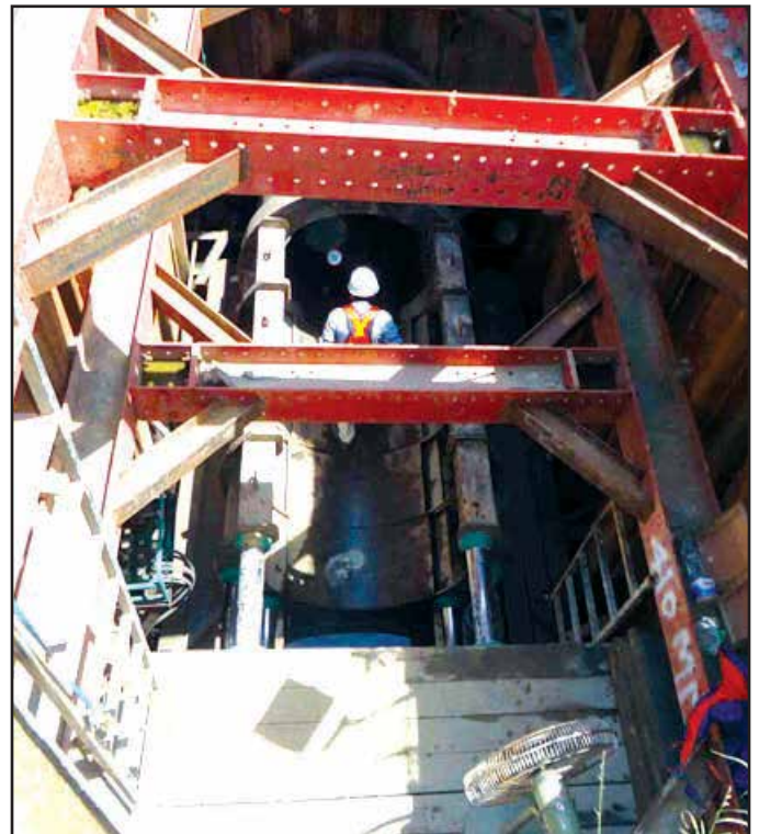
Pipe Jacking at Railway Undercrossing
