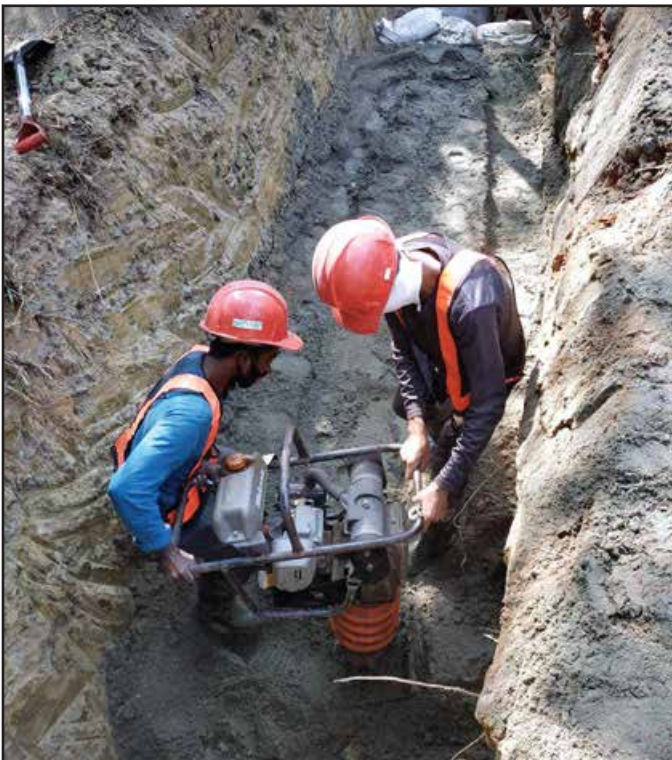
Sand Compaction Work Using Tamping Rammer
