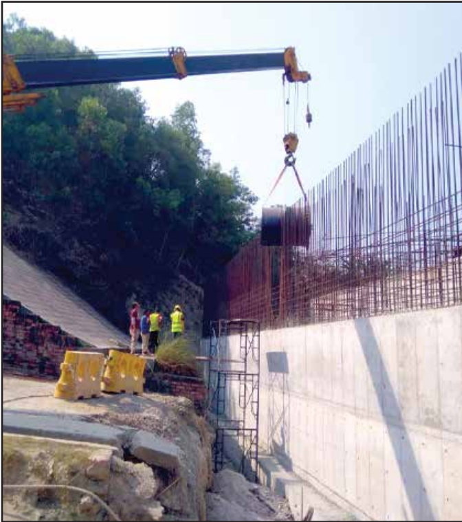
Ongoing Installation of Inlet Pipe
