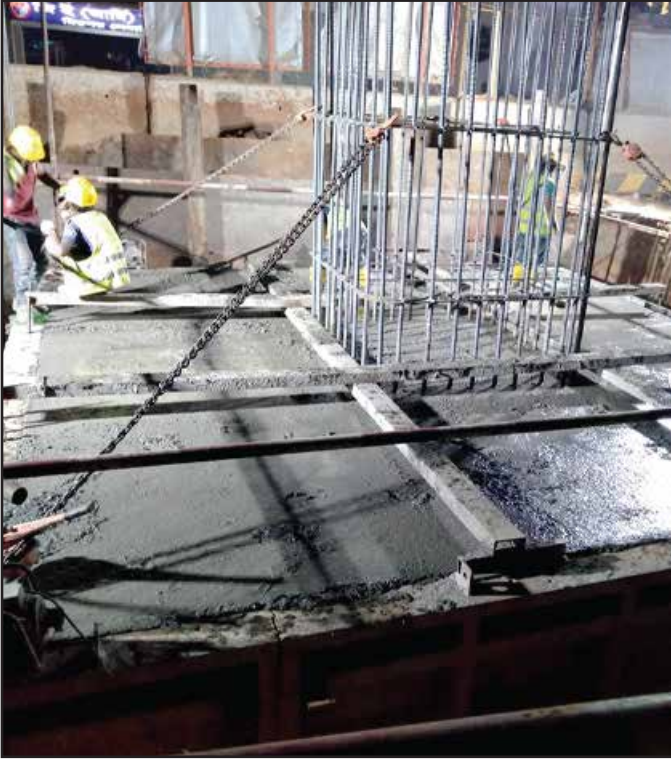
During Pile Cap Concreting
