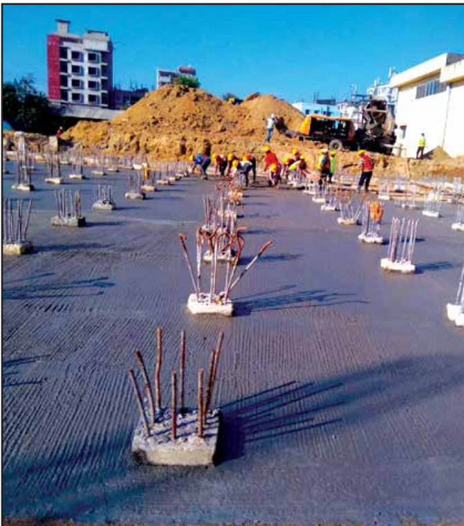
Finishing Work of the Base Concrete
