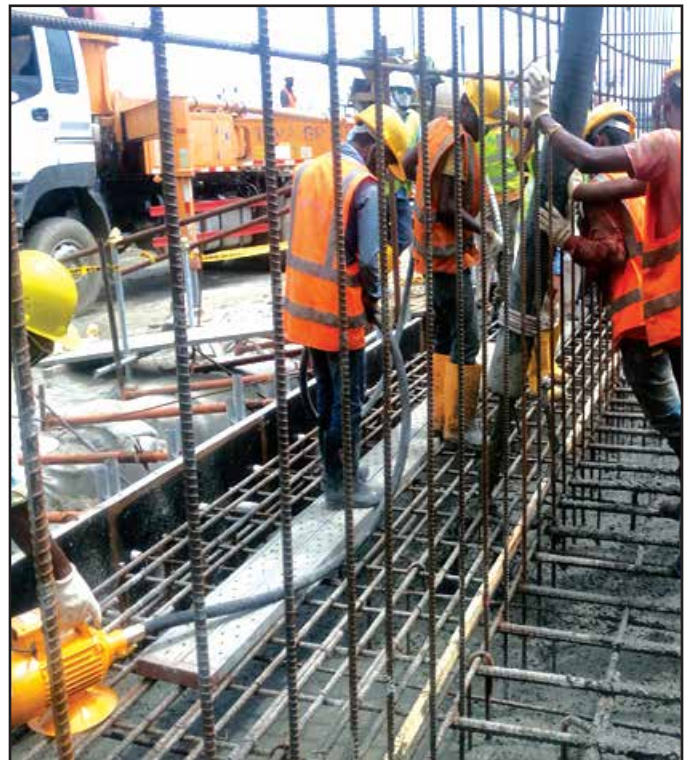
Concreting of Abutment-2
