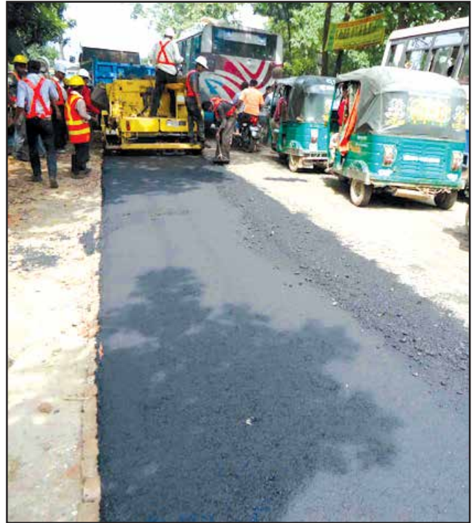
Permanent Reinstatement After Pipe Installation
