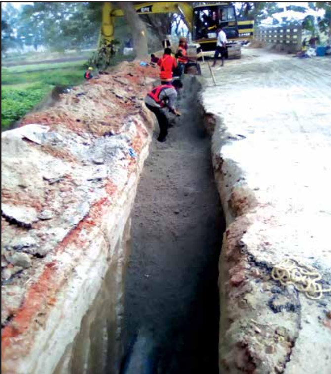
Sand Backfilling Work after Pipe Laying
