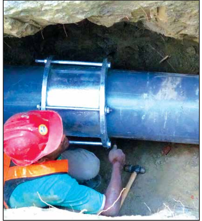
Connecting Dresser between Pipes
