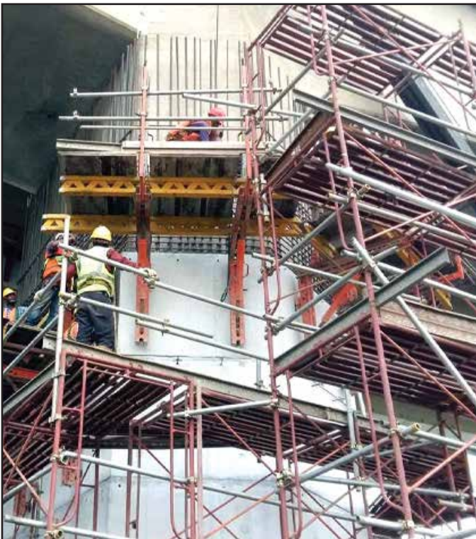
Pier-3 Ongoing Rebar Work (Meghna Site)
