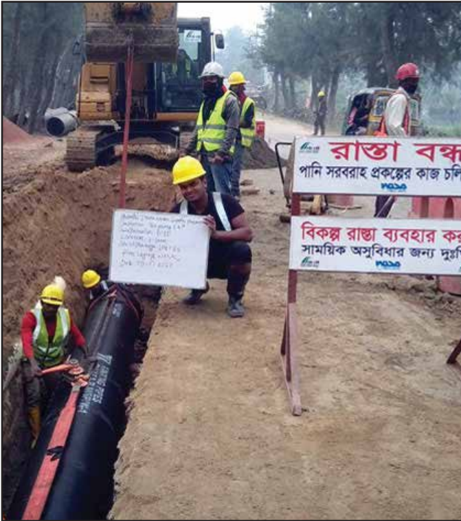
600 mm Dia DI Pipe Laying Work at CUFL Road
