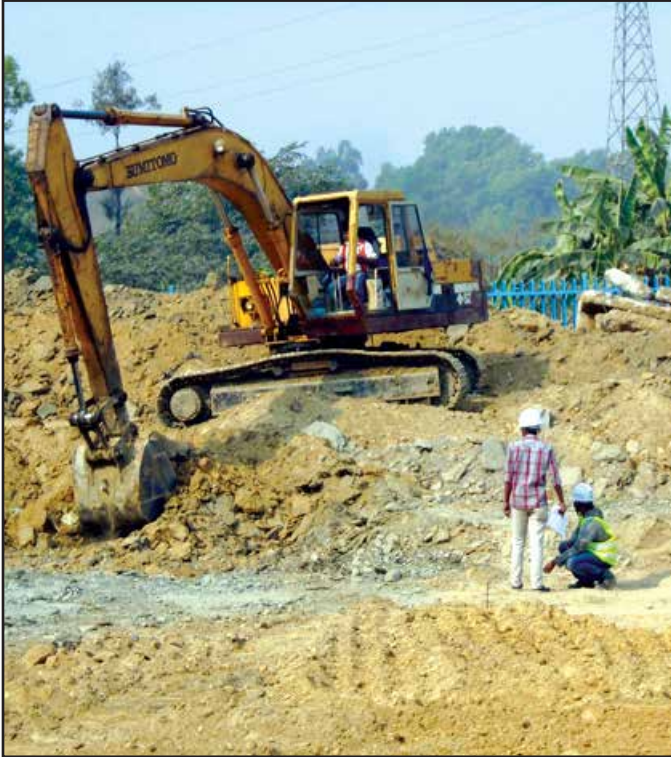
Excavation Work for Reservoir
