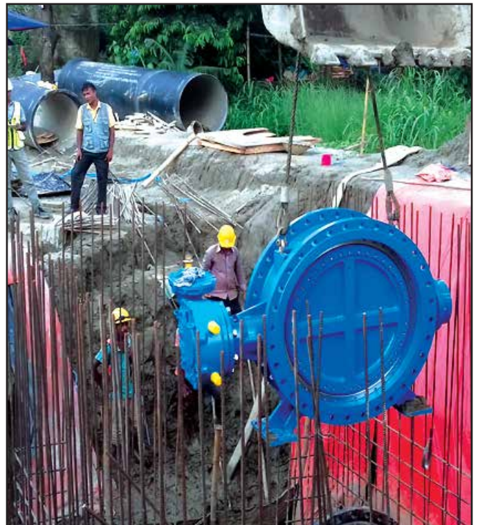
Installation of Air Release Valve in Progress
