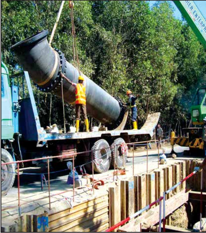
Transporting Pipes to Worksite on a Lowbed Trailer
