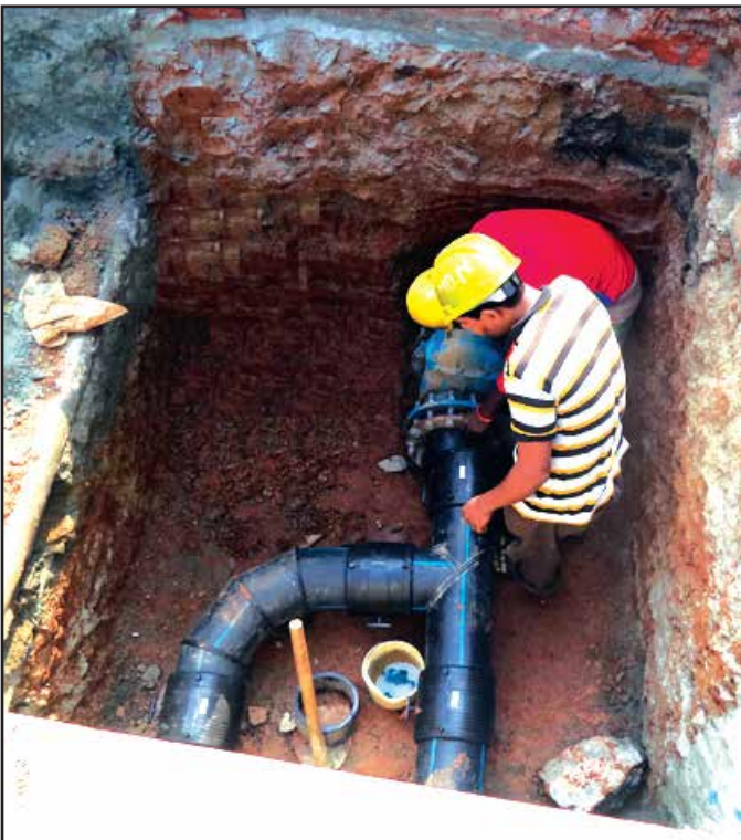
BWM Connection Work
