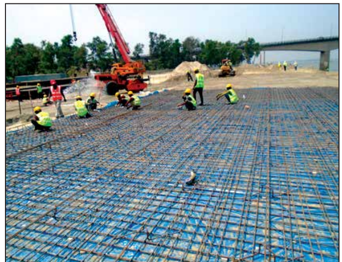
Access Road Rebar Fabrication Work at Jetty Area
