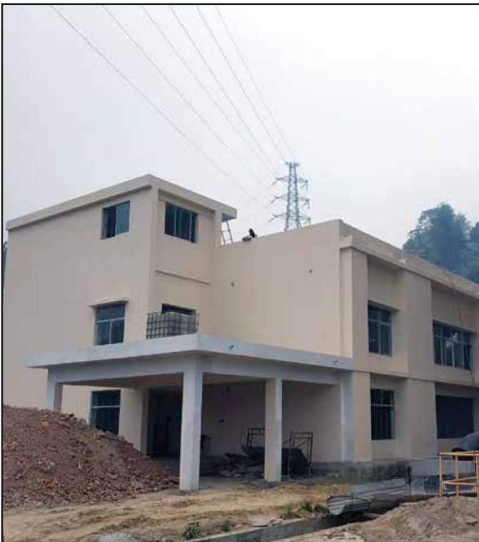
Completed 2-Storyed Water Distribution Management Centre
