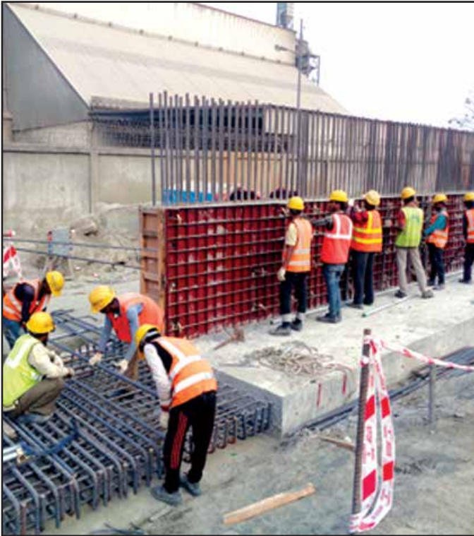
Construction of Retaining Wall
