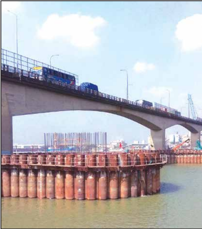
Steel Pipe Cofferdams at Meghna Site
