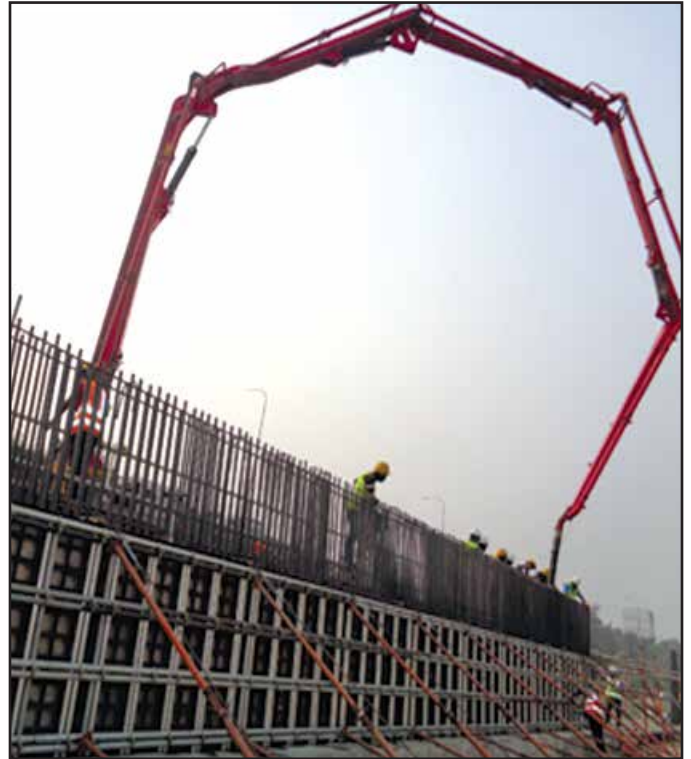
Retaining Wall 1 st Lift Concreting in Progress
