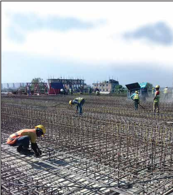
Deck Slab Rebar Work at CP-03 (P16 to P22)
