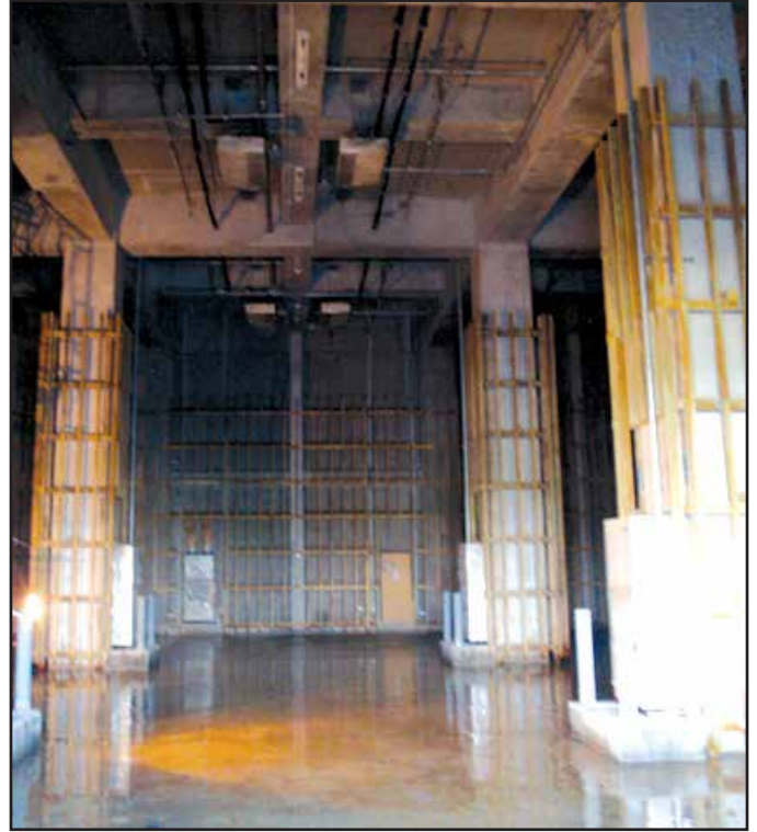
Wooden Lattice on Wall & Around the Columns
