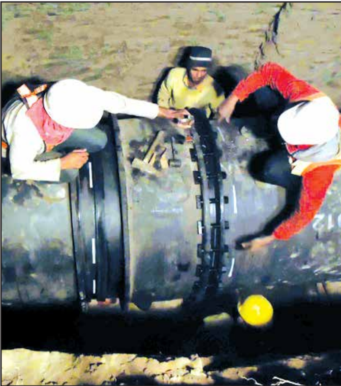
Pipe Laying (TR-1) with Collar Joint
