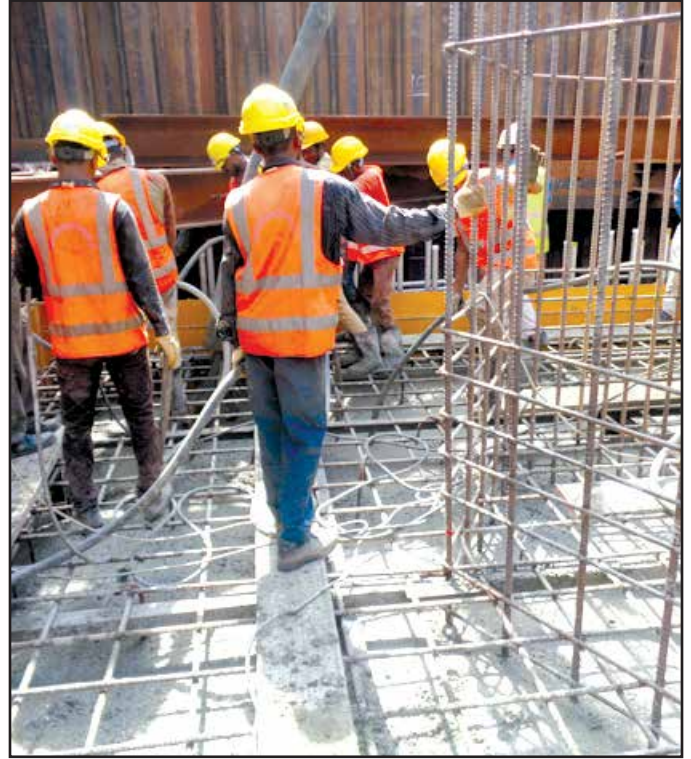
Pier- 11 Pilecap Concreting
