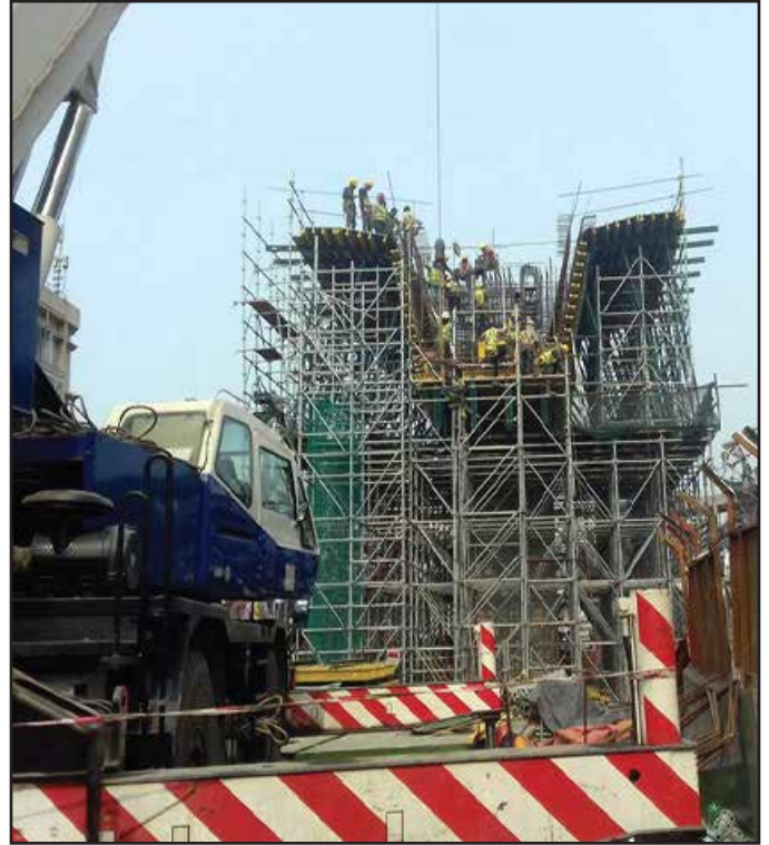
Pier Table Work at CP-04 (P 247 & 248)
