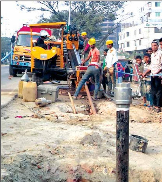
HDD Machine at Work
