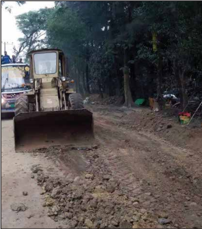
Removing Debris Using Payloader
