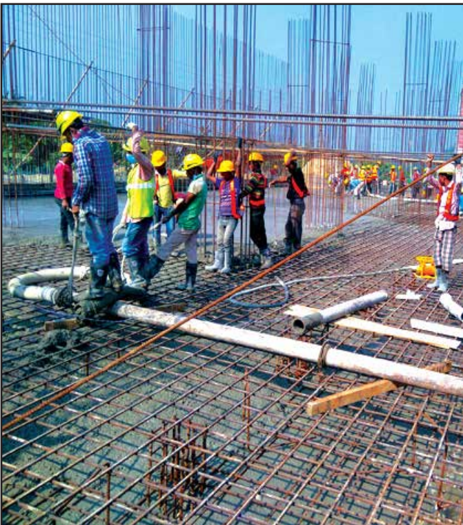
Concreting of Reservoir Base Slab
