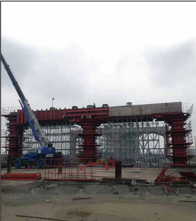
Ongoing Portal Pier Formwork Installation
