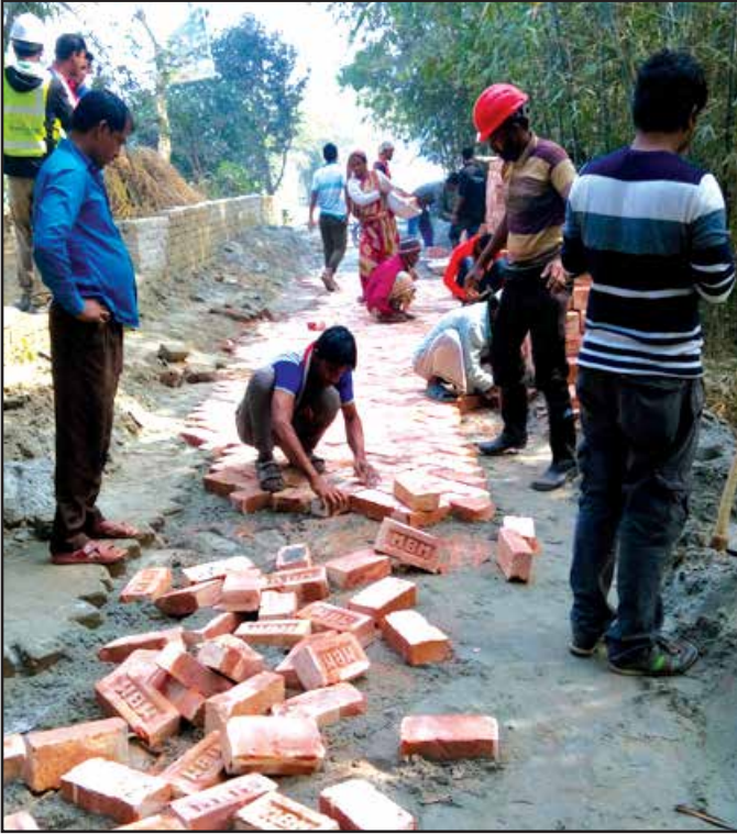
Brick Soling Work in Progress
