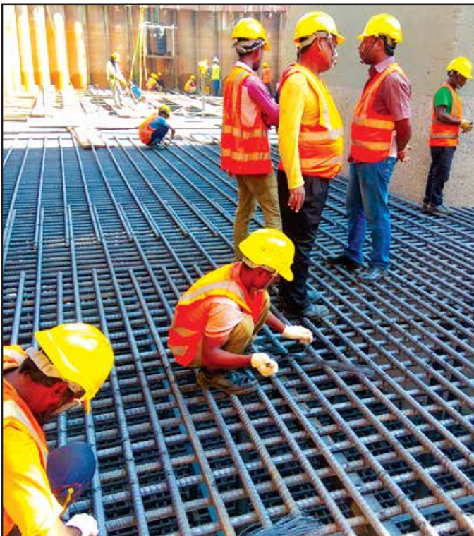
Pier- 10 Final Base Layer Rebar Fixing
