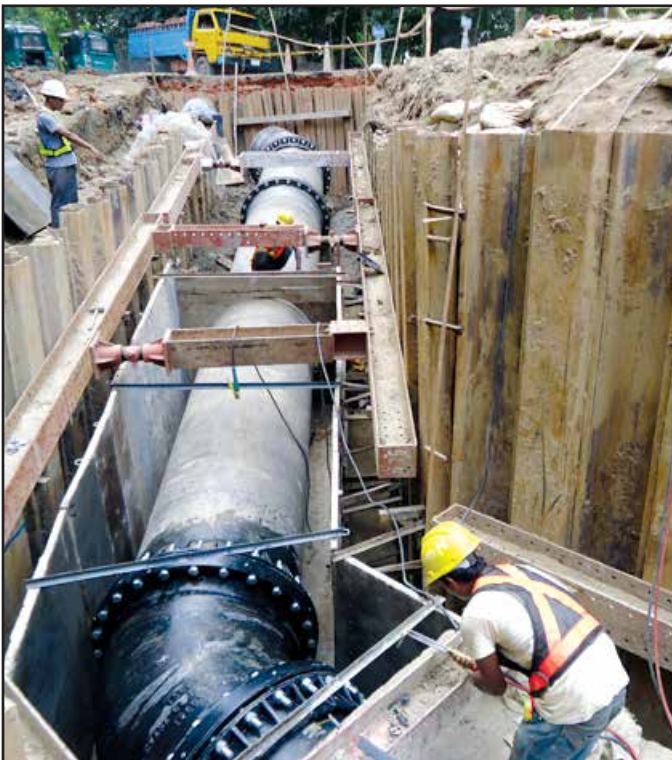
Pipeline Installation using Sheetpile
