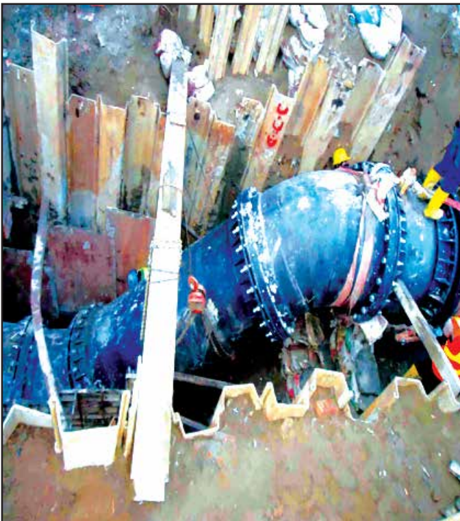
Pipe Laying with Bend (TR-1) & Restrained Joint
