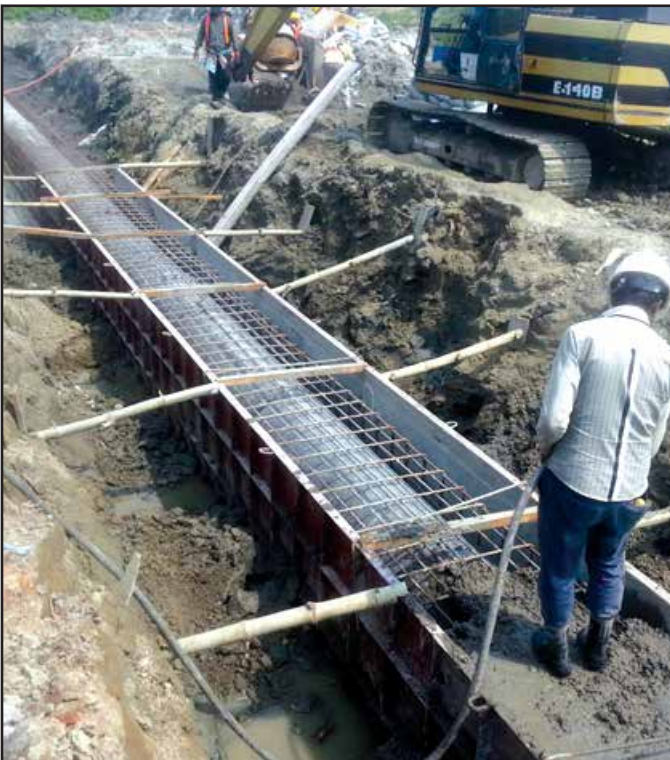
Surrounding Concrete Work in Section-2
