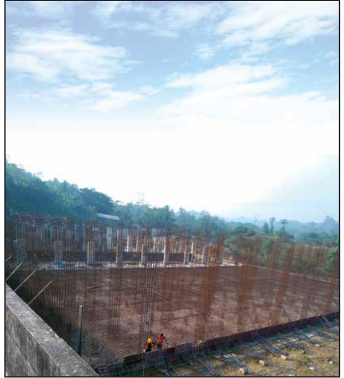
Column Rebar Work for Zone-2 of Reservoir
